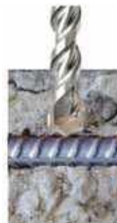
Rebar Step 1 Hammer Drill
