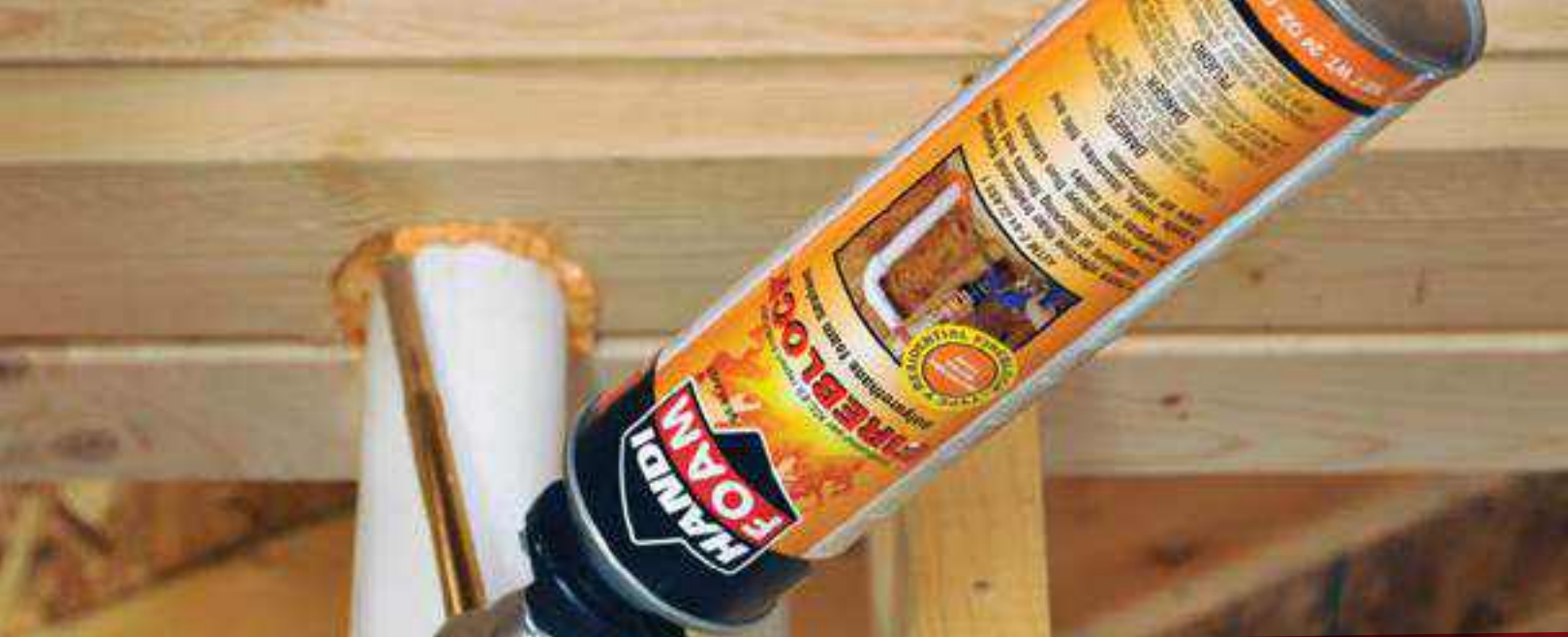
FOR FIREBLOCKING IN TYPE V RESIDENTIAL CONSTRUCTION
