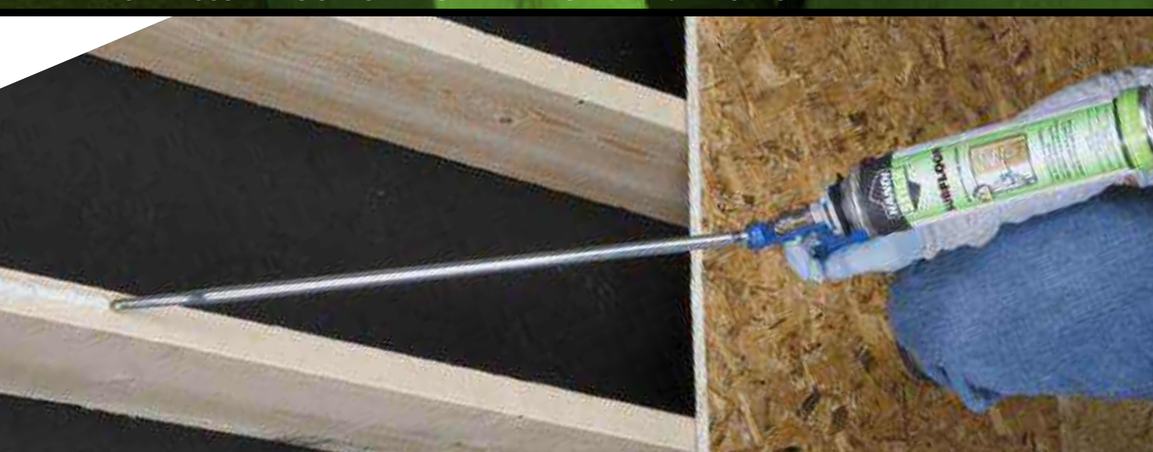
USED IN LAYING SUBFLOOR WITH A 20 MINUTE OPEN TIME
